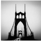
May, 2017 St John's Bridge, Portland, Oregon
